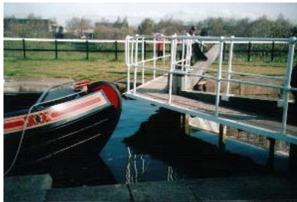
Figure 2.2 Forth & Clyde Canal gates showing overhanging walkways
