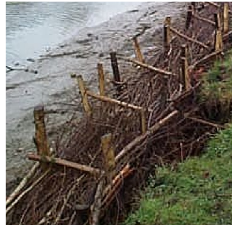
Hazel Faggots being installed
