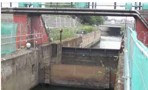
CARPENTERS LOCK BEFORE PARTIAL DEMOLITION
