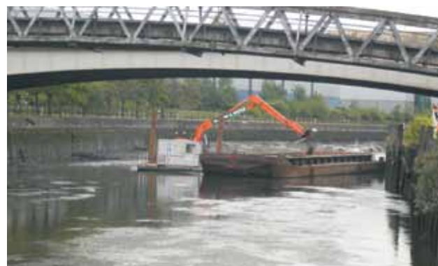
RIVER LEA DREDGING
