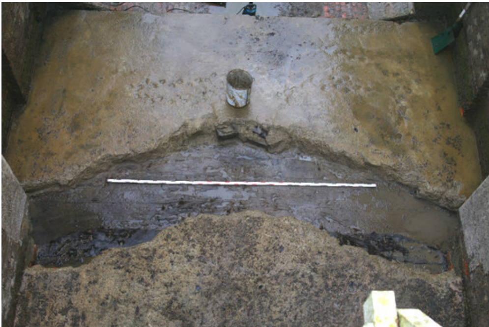
An original timber lock cill archaeologically recorded on the scheduled monument at Caen Hill, Kennet & Avon Canal.
