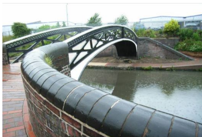
A Grade II listed roving bridge on the BCN at Bromford Junction, repaired in 2007.
