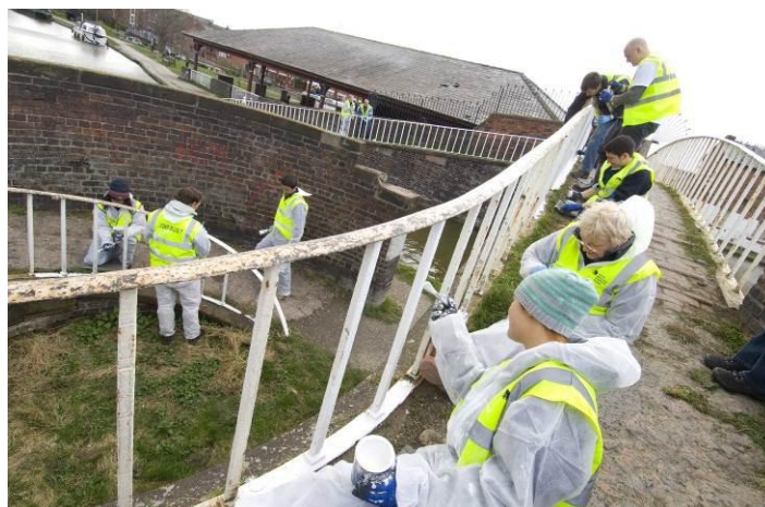
Volunteers repainting the turnover bridge at Tower Wharf, Chester
