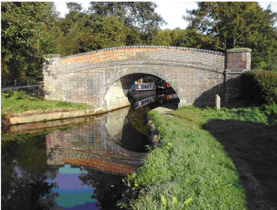
Willow Cottage Bridge, Caldon Canal – heritage repairs won a national Highly Commended Prize in 2010.
